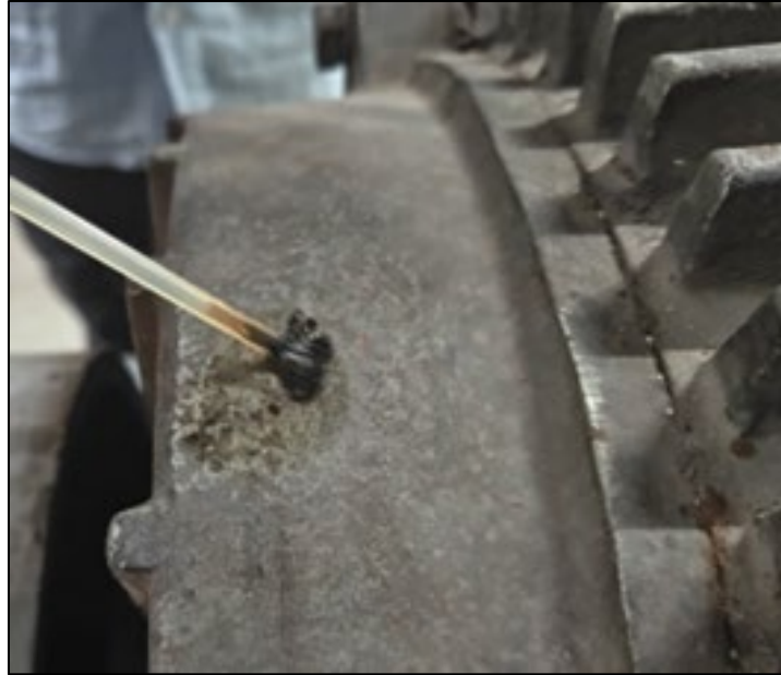
Figure 7: Activator applied on surface
